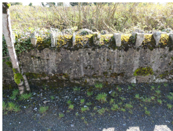
Fig.15 Section 05, mass concrete repair
