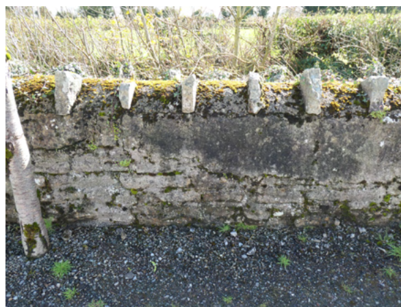
Fig.13 Section 03, mass concrete repair
